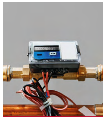
Smart water meter
